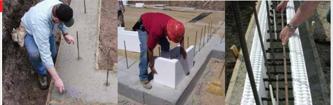
1 Prepare the job site
