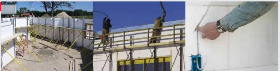
4 Brace the wall
