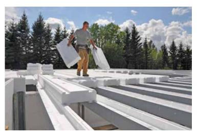
value of EPS rigid insulation and the added structure and flexibility of metal cladding. Fortruss perfectly compliments your Insulated Concrete Form (ICF) structure and together they provide a complete structural and thermal "building envelope".
