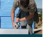
3 TRUSS FORMS CAN BE EASILY CUT AND MODIFIED ON SITE.
