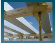
ONCE TRUSS FORMS ARE IN PLACE, SIMPLE SHORING IS ERECTED.
