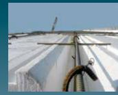
6 REBAR AND STIRRUPS ARE THEN PLACED ACCORDING TO DESIGN SPECIFICATIONS.
